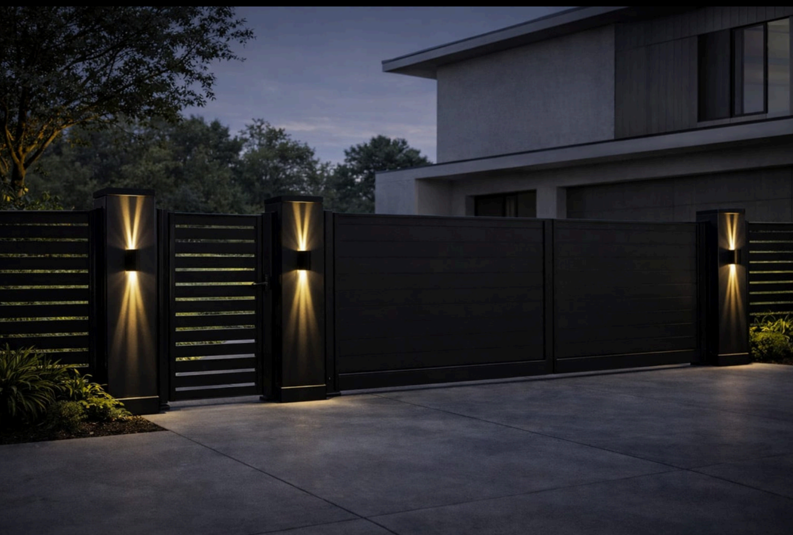
Double Door Gate • Installed
